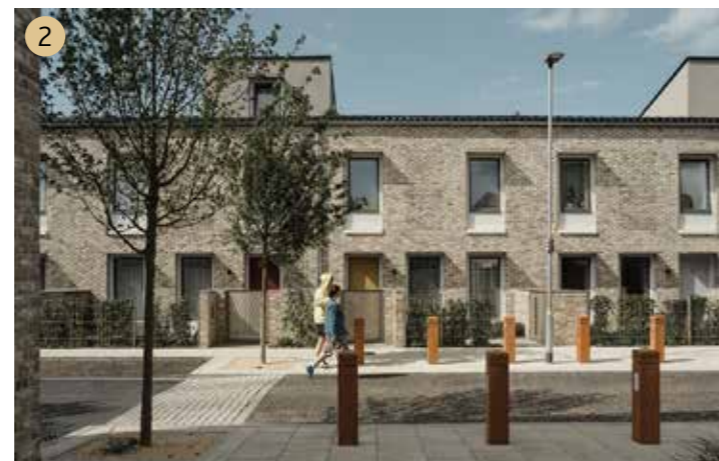
Contemporary terraced neighbourhood - Goldsmith Street, Norwich (Image Credit: Tim Crocker)
