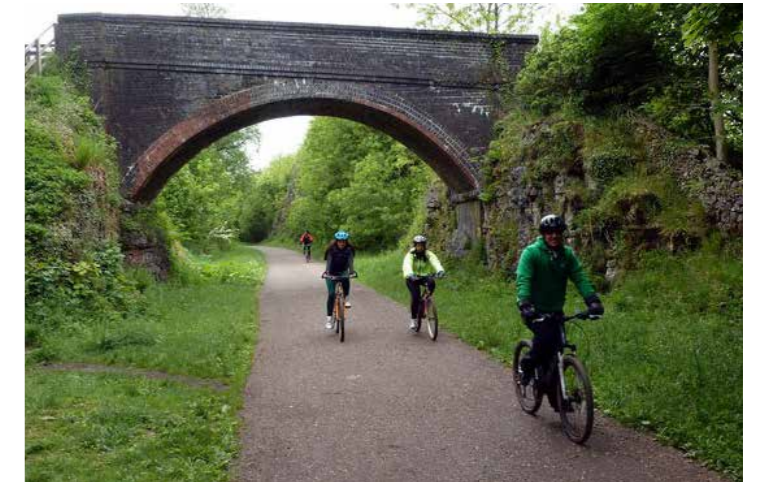
Active travel link in natural landscape through historic arch
