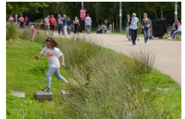
SuDS Swales integrated with GI and active travel routes provide green links across the site
