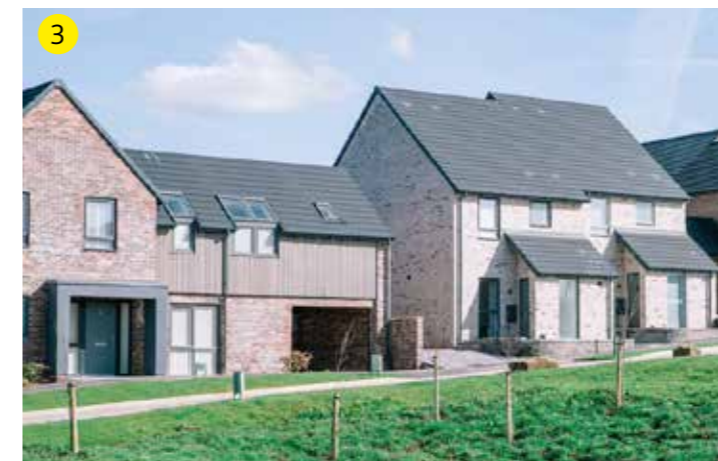
Local brick family housing responding to topography - Greenhills, Blackburn
