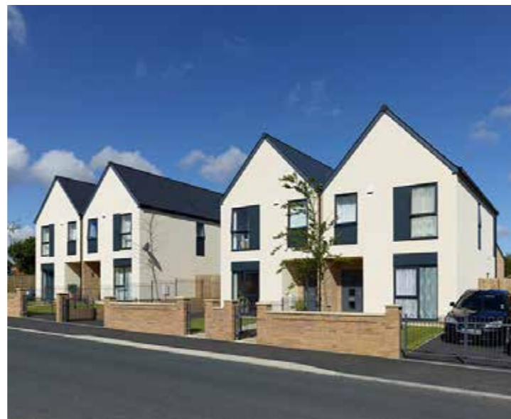
Precedent of residential frontages and appropriate setbacks from a tertiary street - Madeley Rd, Wakefield
